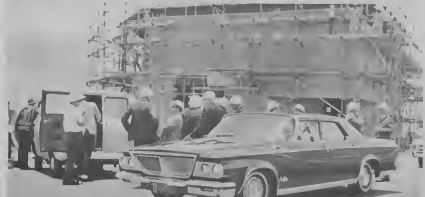
MEMBERS OF Administrative Council stop at new Oil Movts. Controlhouse now under construction.
